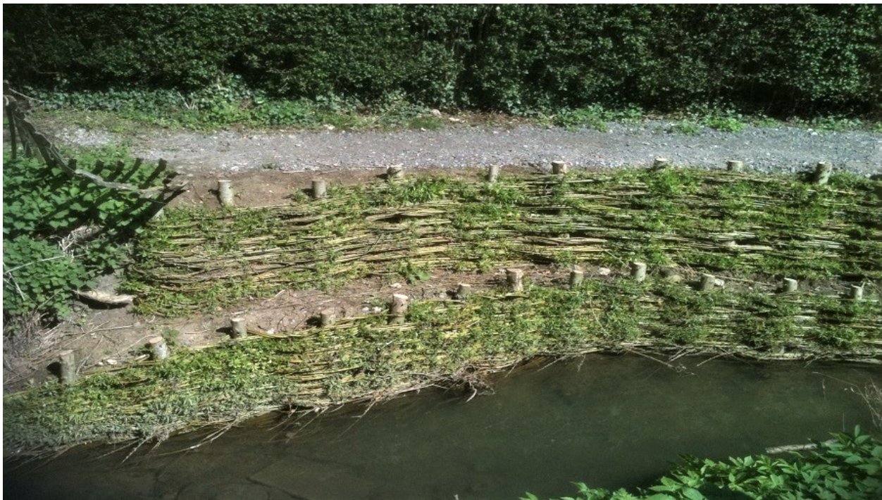
Figure 4. Example of a Willow Revetment
